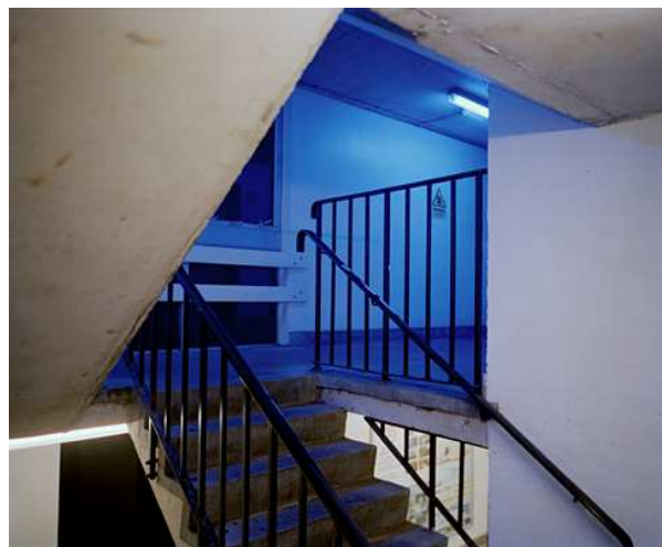
Level 1 stairwell, King Place car park, Brighton, UK.
